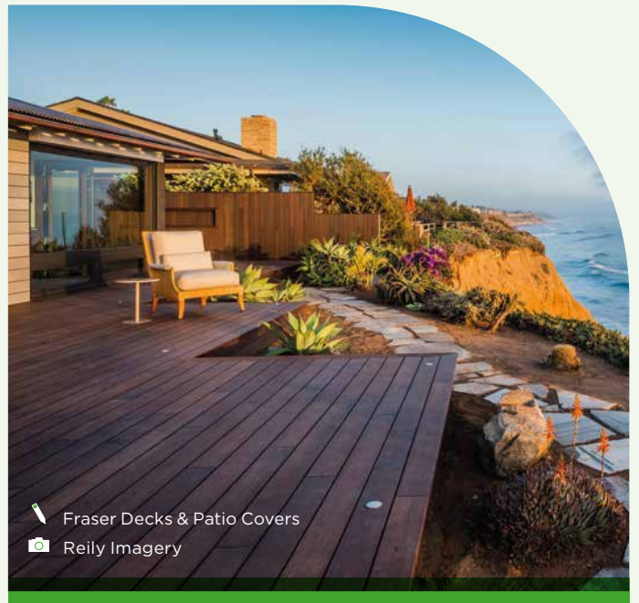
Private Residence Solana Beach low clearance decking installed near a cliff edge by the sea - (325 m 2 ) California, USA
