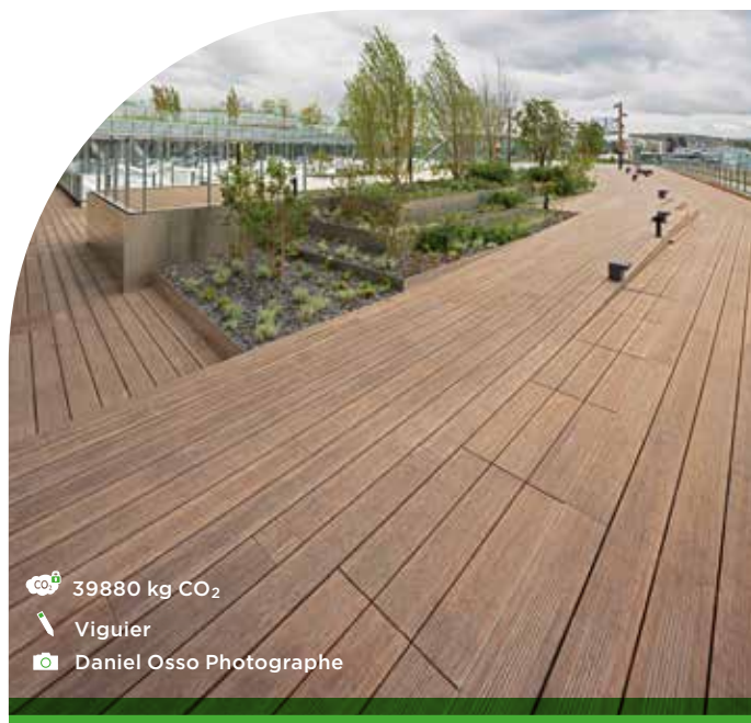
Bridge Pont d'Issy Orange Head Office (1200 m 2 ) Issy-les-Moulineaux, France
